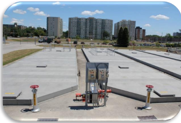
2000 - Flat Covers installed at the London WWTP
