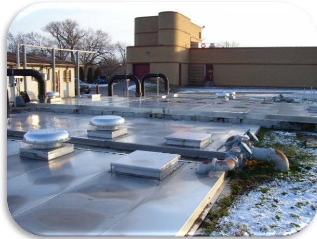
2003 - Flat Covers installed for Caledonia, Haldimand County.
