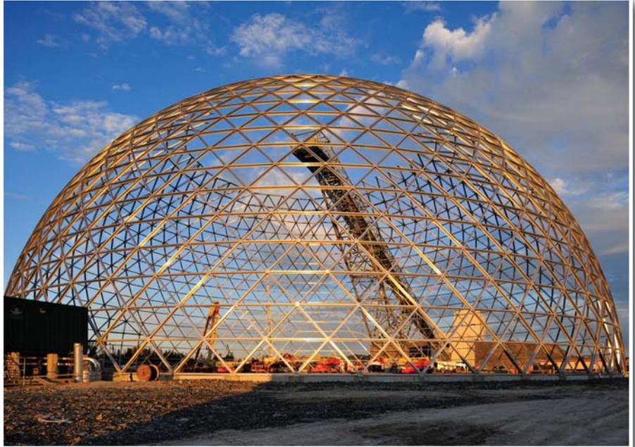
*In total, 3,363 beams were constructed into aluminum gussets to form the structure. Photo courtesy Detour Corporation and Graeme Oxbly.*
