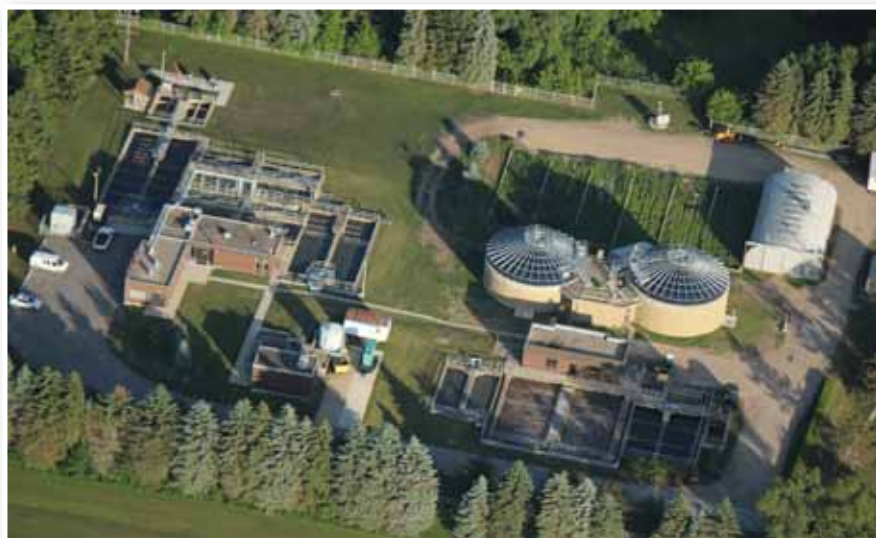
Aerial view of the Ingersoll Wastewater Treatment Plant.
