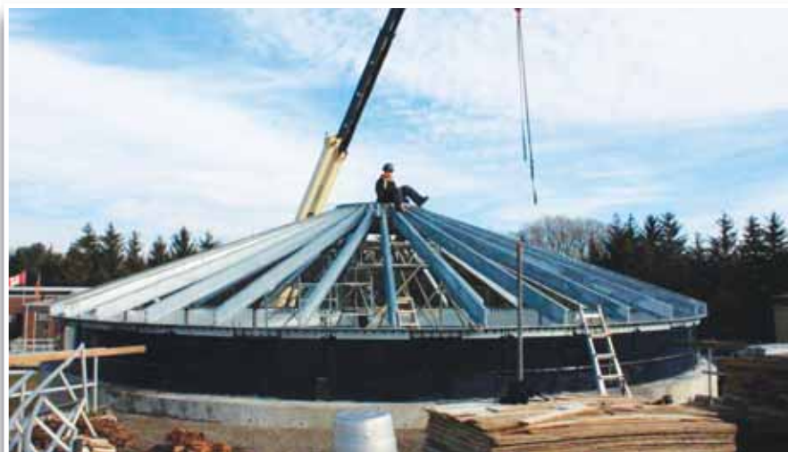
Greatario's externally supported roof is built to accommodate higher static and dynamic loads.
